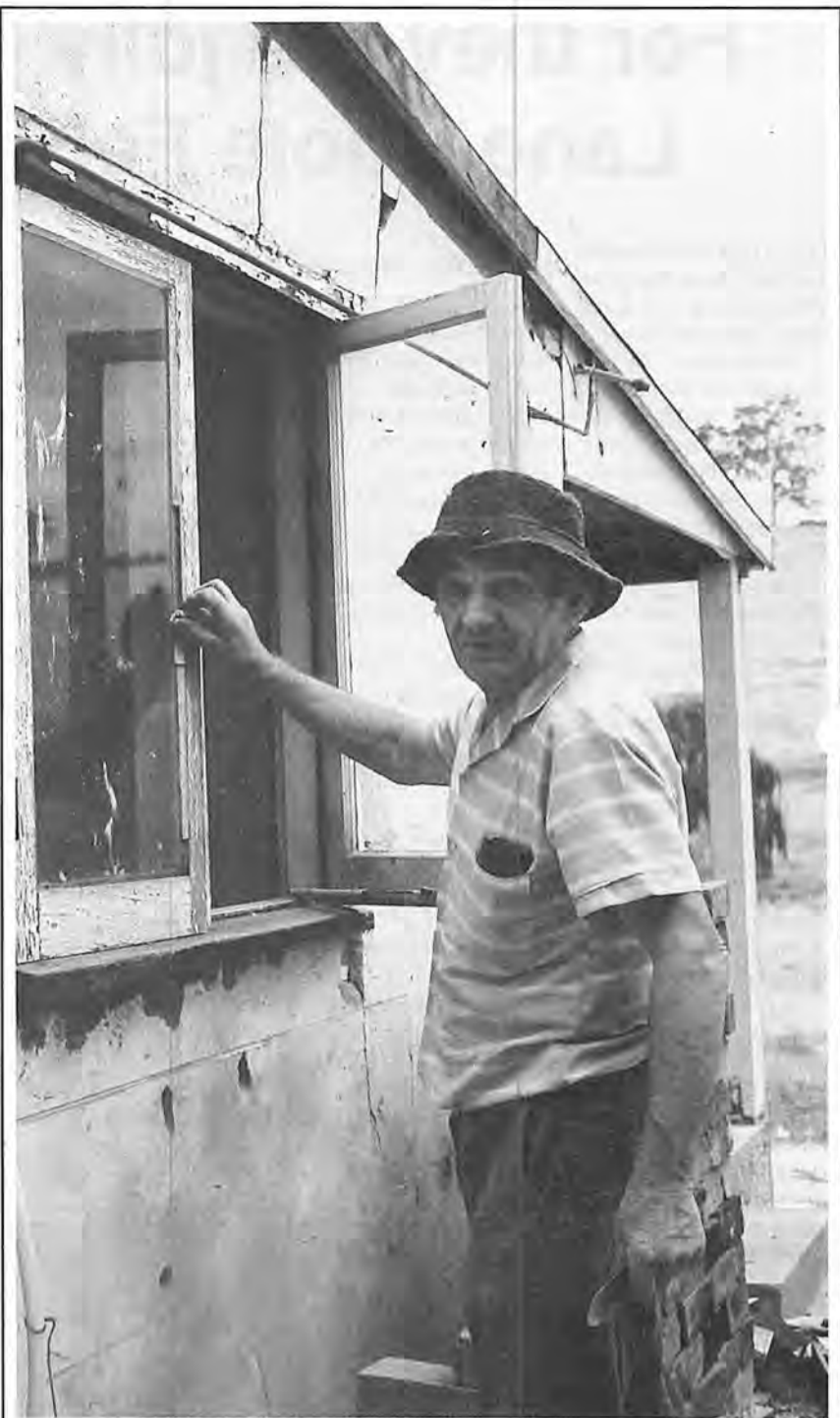
Technical advisor Helmut Hiddel checking glazing work at the homestead. Photo by Carolyn Thomson
