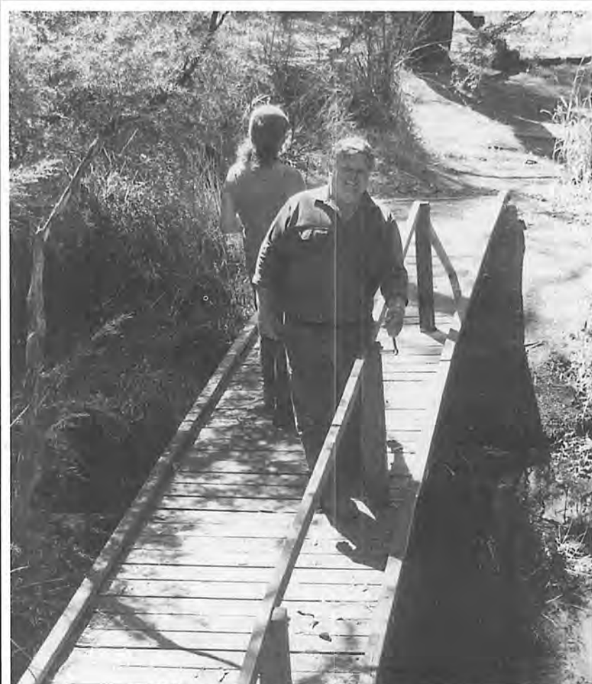
After waiting for shrinkage of the green wood to occur, forest workers Keith Harris and a camera-shy Kevin Pratt check the stability of one of the Lane Poole Reserve bridges. Photo by Tammie Reid
