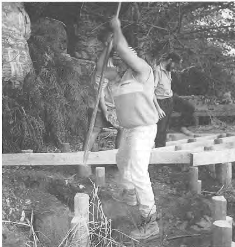
Laying down stumps and bearers for the boardwalk and viewing platform at Fern Pool are, left to right, Adrian Lawson, CEPANCRM leading hand Phil Young, and Joseph Limerick. Photo by Johnny Parker
