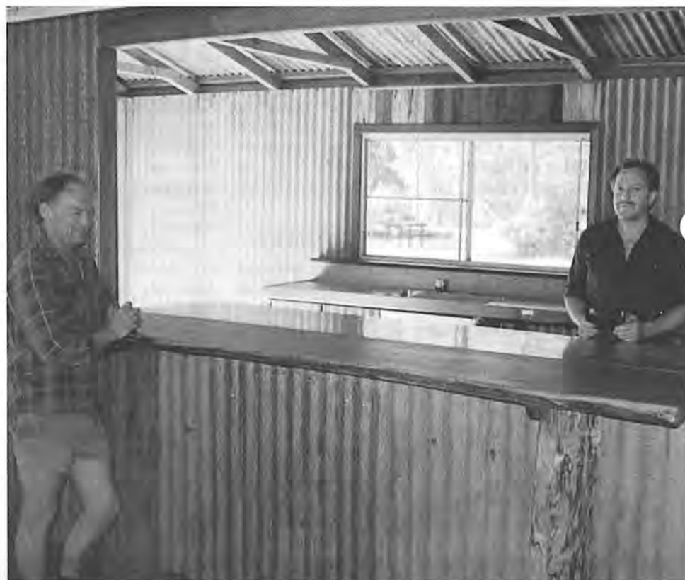
Forest workers Mal Strange (left) and Anthony O'Neill reflect on their craftsmanship after completing the bush kitchen. To give a rustic look, second-hand corrugated iron was used for internal and external cladding. Photo by Glenn Willmott.
