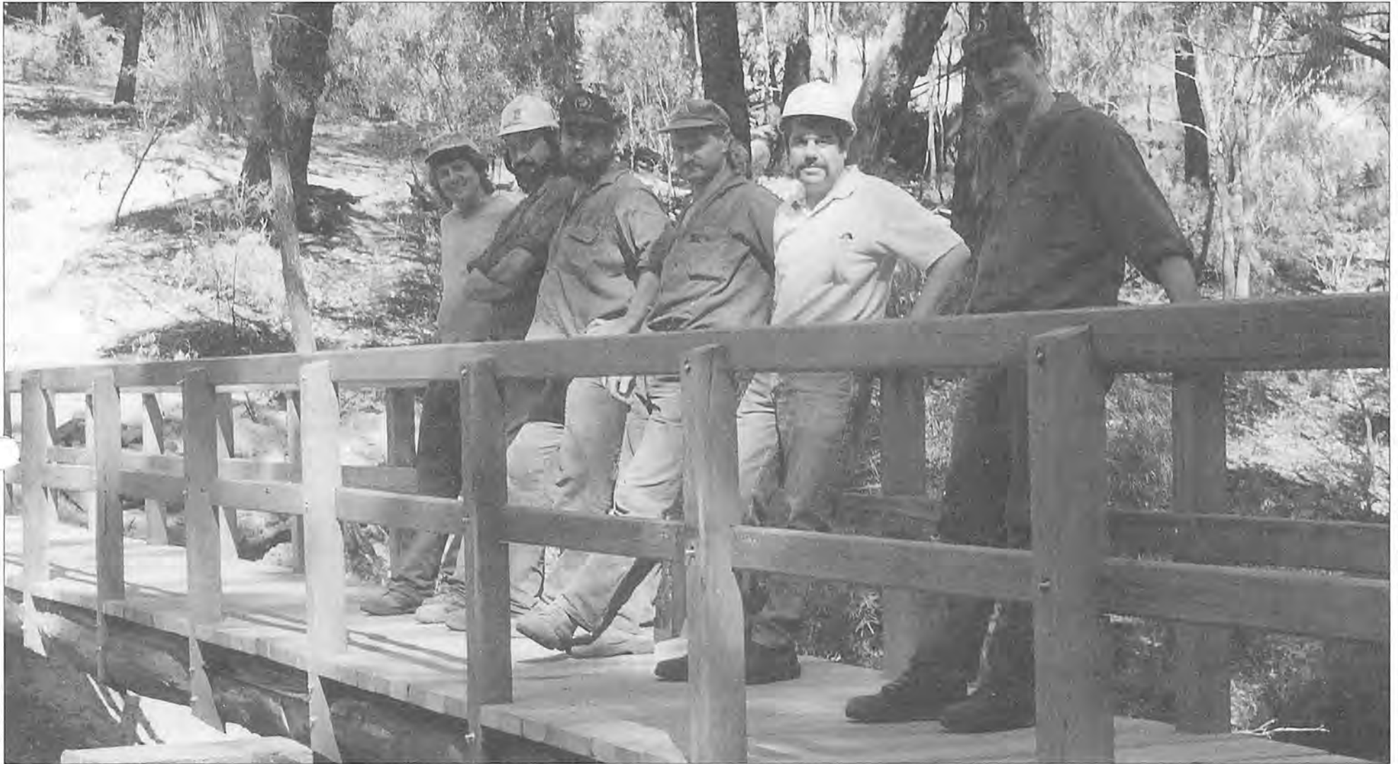
Left to right: CALM forest workers Michael Liebrechts, Peter Beebe, Sid Sepkus, George Laws, District manager John Gillard, and overseer John MacDonald. They are on the 24-metre-long bridge across Gardner River, south of Northcliffe. Photo by John Gillard
