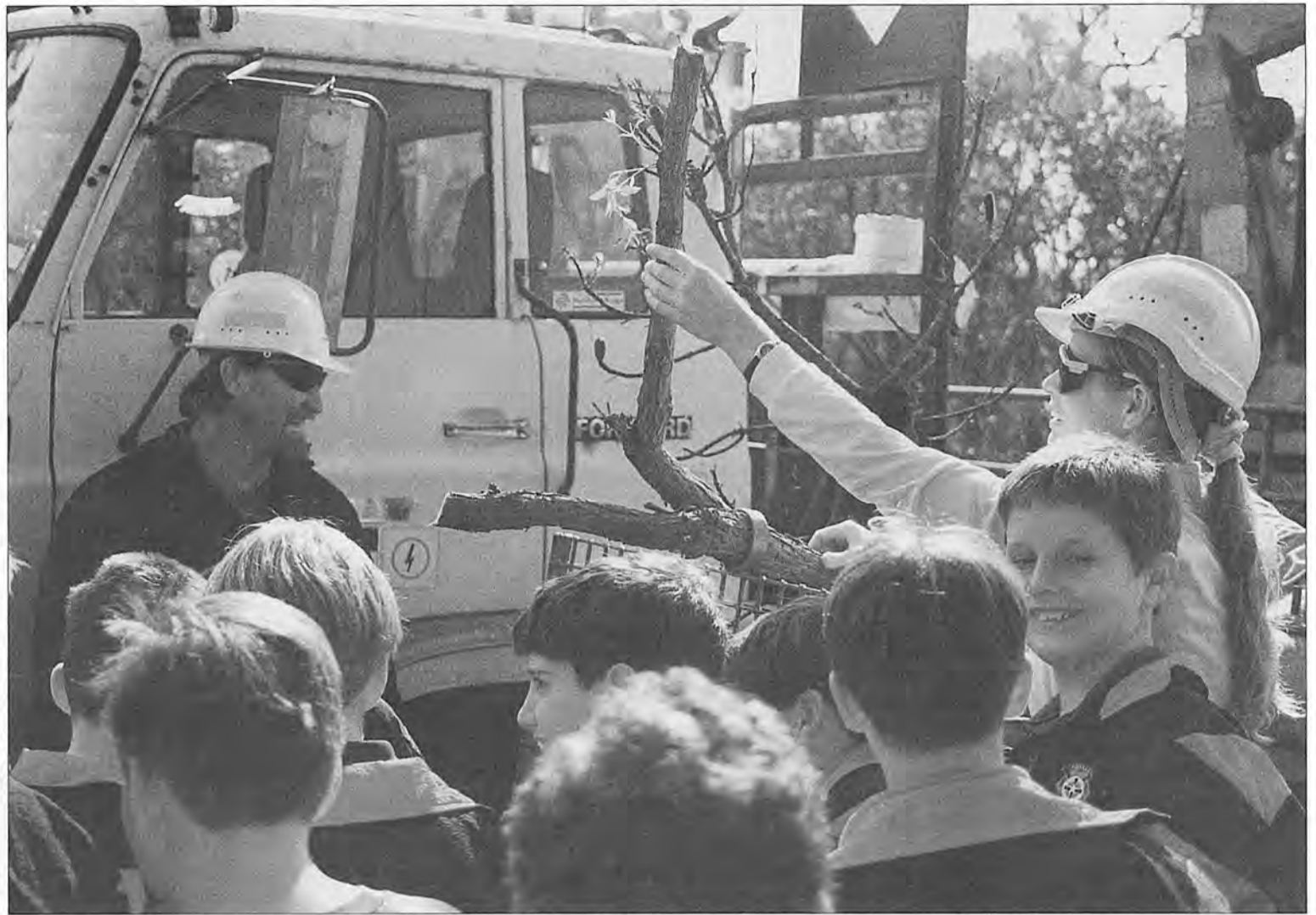
Land for Wildlife administration officer Emma Bramwell (far right) and Aquinas College students William Harfield (next to Emma), and Luke Fiorentino (centre) with unidentified classmates, help Western Power's Neil Smith with the installation of an osprey nesting platform. Photo by Rachel Nordeck, courtesy Aquinas College
