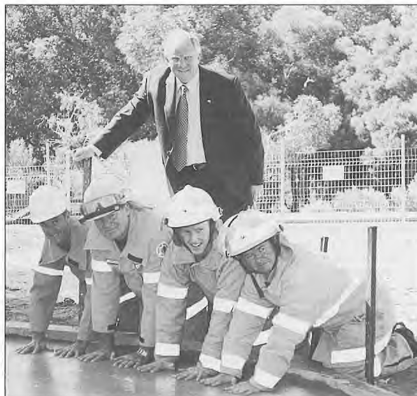
Four firefighters 'handprint' wet concrete foundations of the Firefighters' Memorial. They are (from left) CALMfire crewman Doug Giles, Parkerville Volunteer Bush Fire Brigade captain Laurie Hudson, Perth Fire and Rescue Service, career firefighter Nathan Boothman, and Secret Harbour Volunteer Fire and Rescue Service captain Kevin Archer. Looking on is Emergency Services Minister Kevin Prince.
