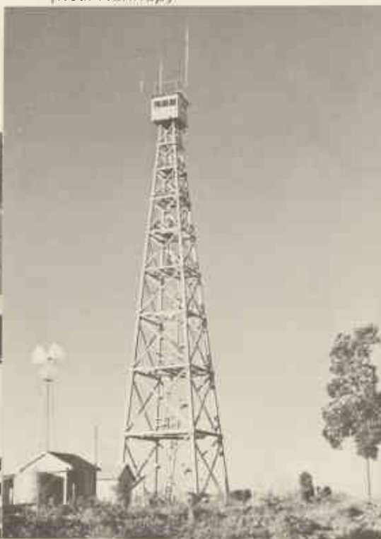
Repeater station combined with fire lookout tower (near Nannup)
