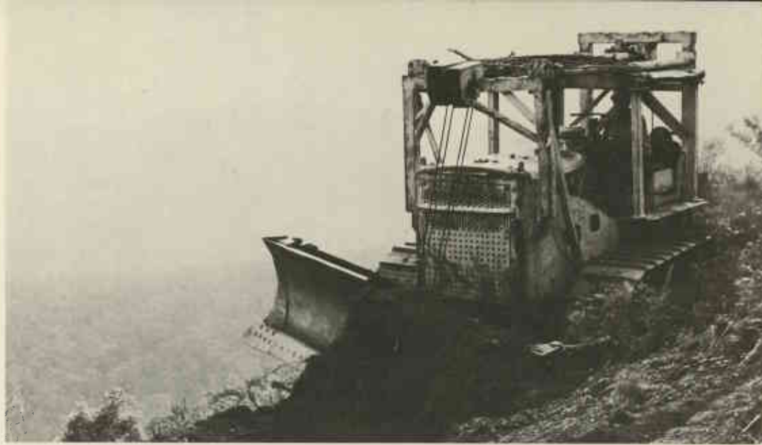
Preparing contour road in steep country (above).
