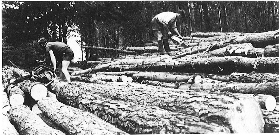
Contractor's employees working at log dump, Milward thinning operations (above).
