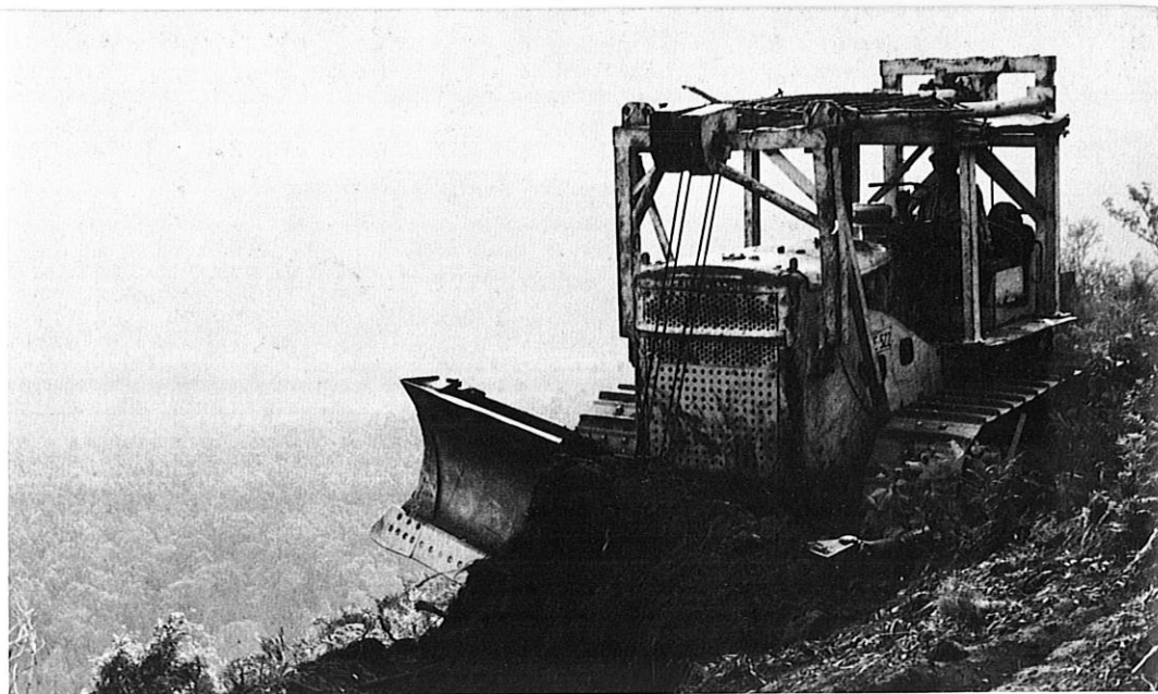
Preparing contour road in steep country (above).
