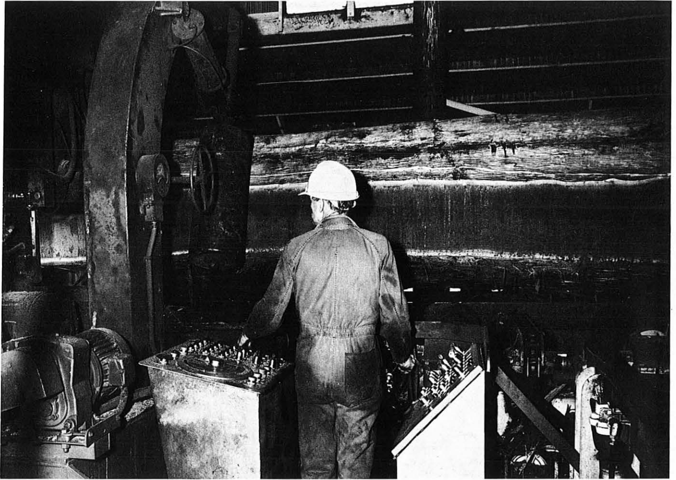
▲ Push-button operated bandsaw log breakdown unit at Lloyds Lumber Co., Greenbushes.
