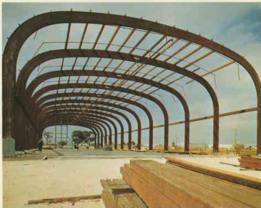
▲ Two examples of timber used for structural purposes. Above, termite-proofed pine framing and roof timbers of a semi A-frame home at Australind, built by F. and L. M. Burke. Below, the huge new Bunnings building at Welshpool, supported by 705 by 127 mm glue laminated jarrah arches and spanning 19.5 m. The building is 110.95 m long with 8.53 m maximum internal height.
