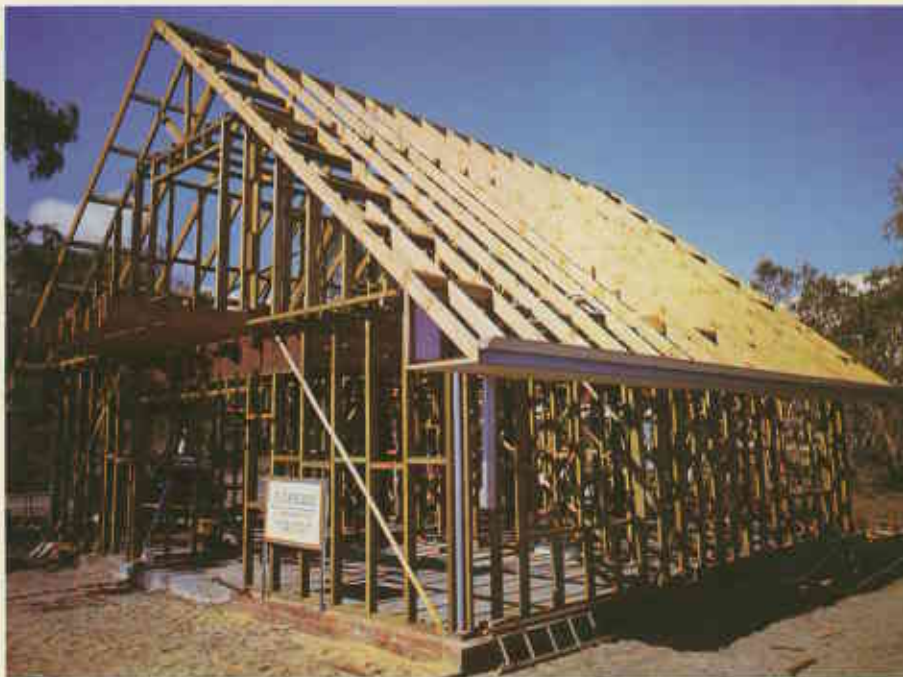
▲ Two examples of timber used for structural purposes. Above, termite-proofed pine framing and roof timbers of a semi A-frame home at Australind, built by F. and L. M. Burke. Below, the huge new Bunnings building at Welshpool, supported by 705 by 127 mm glue laminated jarrah arches and spanning 19.5 m. The building is 110.95 m long with 8.53 m maximum internal height.
