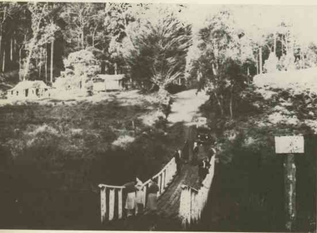
▼ The redecked bridge—note the more sophisticated bridge timbers and also the more delapidated smaller house in the background. Tourists from two cars are admiring the scenery.
