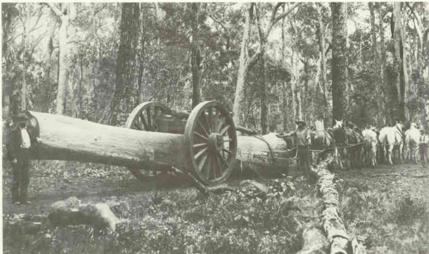
▼ The log winched up into the whim. Note how the leading end of the log acts as a brake on the ground when the team is stationary.
