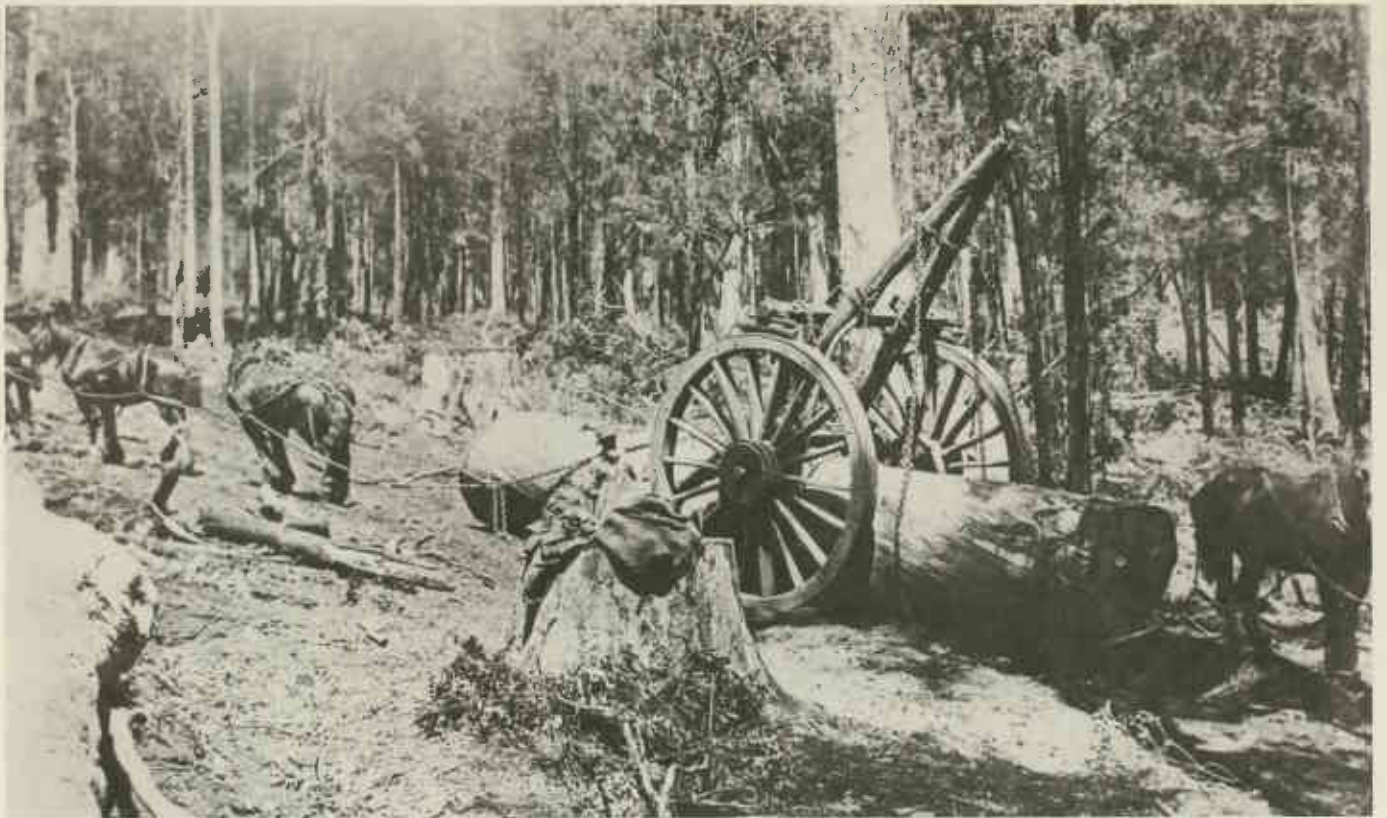
▲ To load the log, some of the horses were used to drag the whim backwards over the log.
