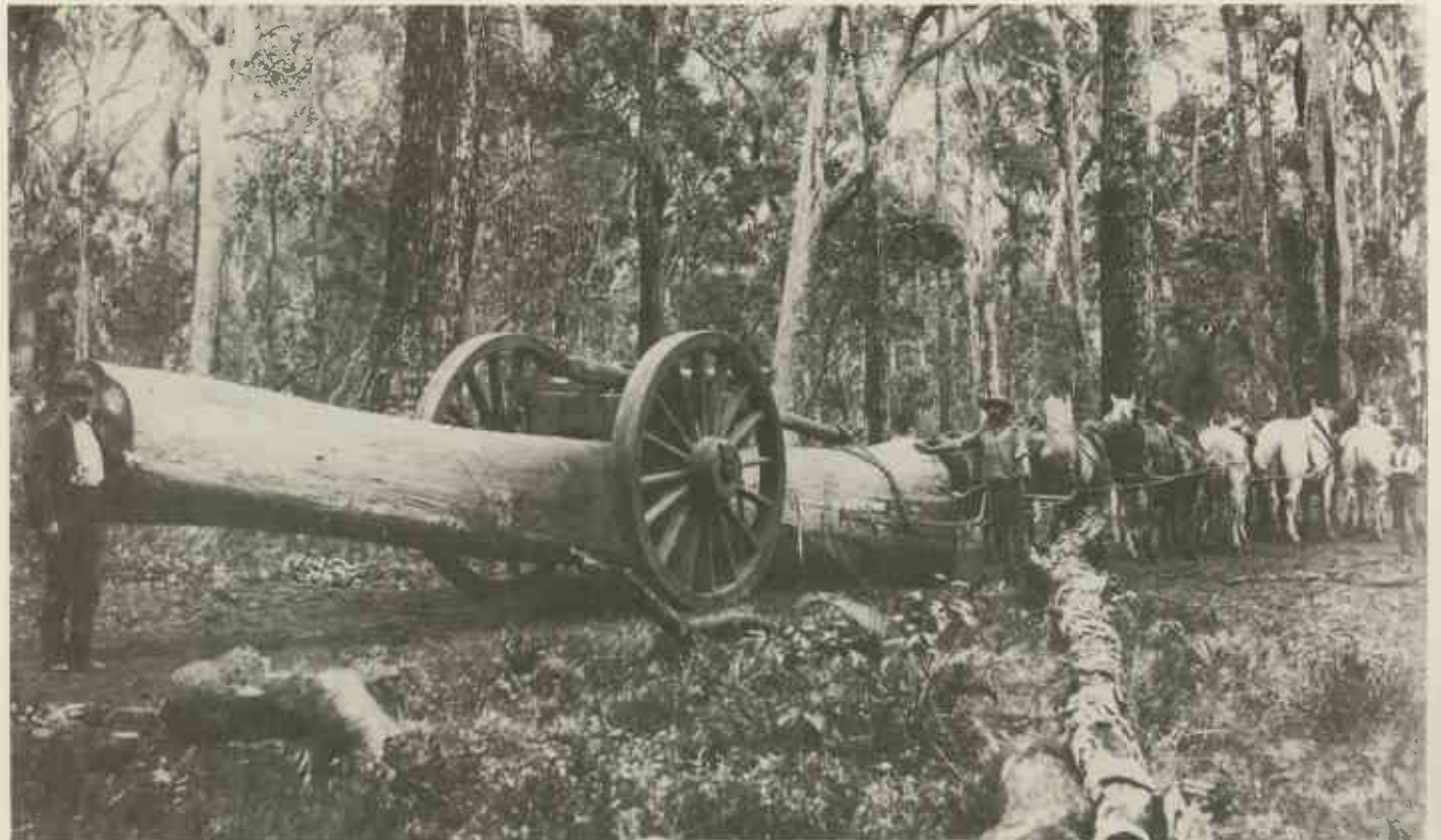
▼ The log winched up into the whim. Note how the leading end of the log acts as a brake on the ground when the team is stationary.
