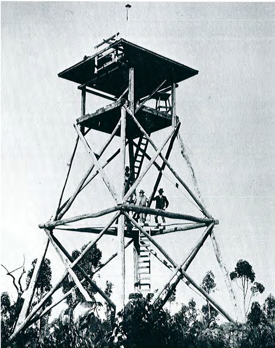
◀ The original Mt. Gungin fire lookout tower built in 1921 and situated some 6.5 km south-east of Mundaring Weir. The towers on Mt. Gungin and Mt. Dale (1921) were the first built by the department. (Anon.)
