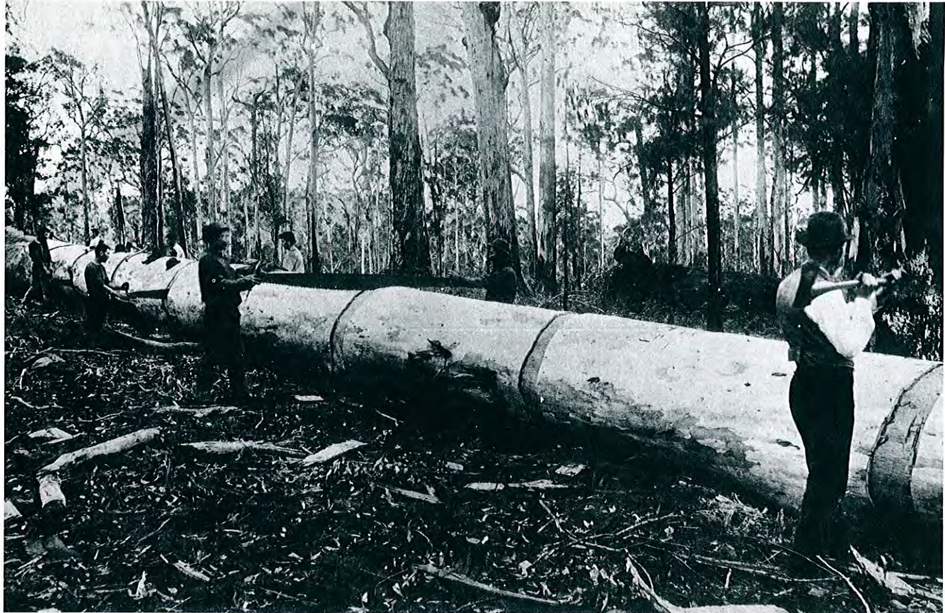
▲ Cross-cutting karri log (working up from the stump end) ready for snigging to log landing.
