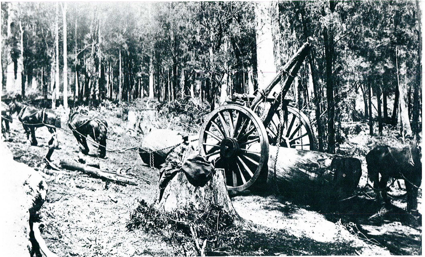
▲ To load the log, some of the horses were used to drag the whim backwards over the log.
