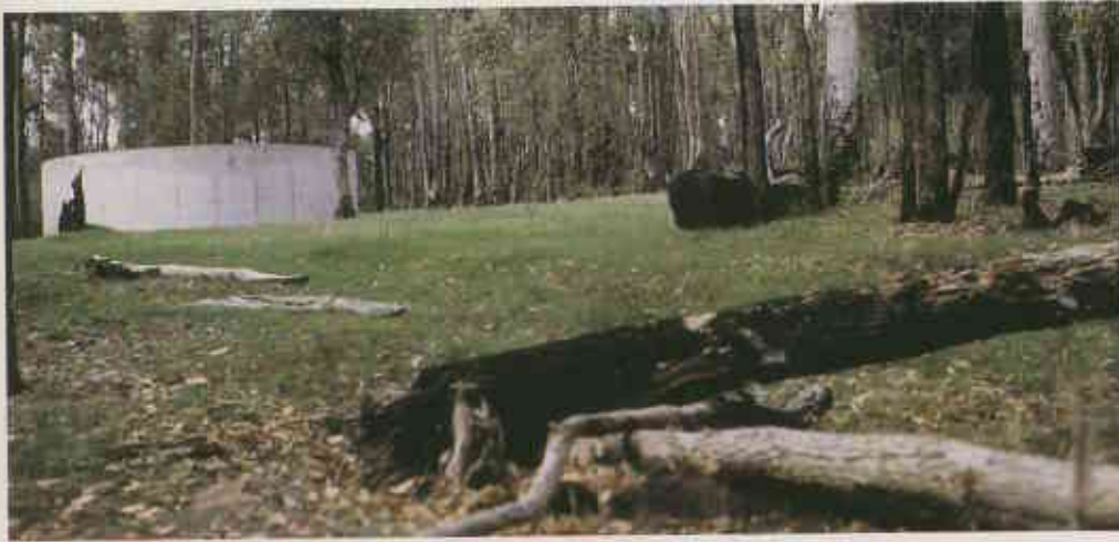
▲ One of the few improvements in the wooded section of "Tanglewood" has been the construction of this water tank holding approximately 50 000 litres. (C. Pead)
