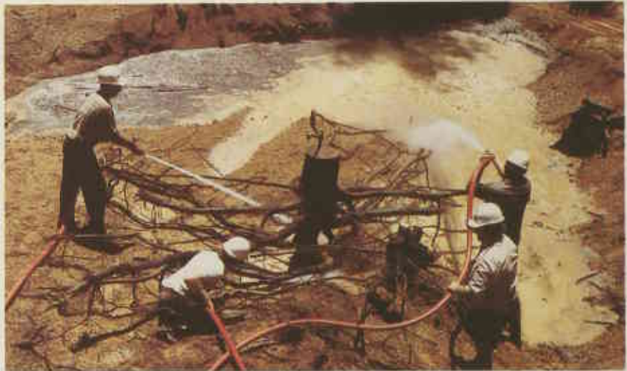
▲ Forests Department fire tankers, supplied with water from large tankers provided by Alcoa, were used for the hydraulic excavation of root systems.
