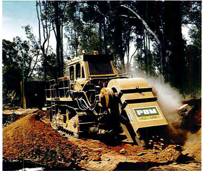
▲ This giant 'Rocsaw', provided by ALCOA, was used to cut sections through the soil profile on severely diseased sites in an attempt to identify the characteristics of the laterite layer.
