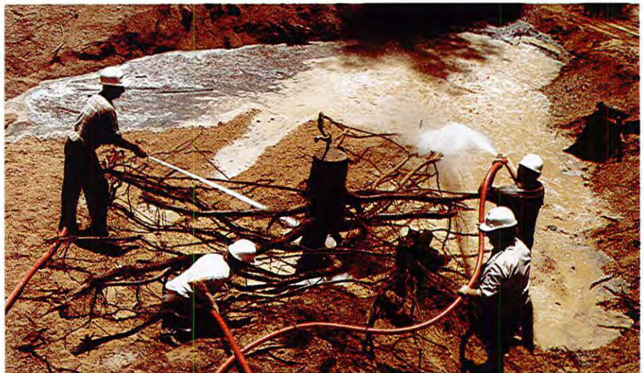
▲ Forests Department fire tankers, supplied with water from large tankers provided by Alcoa, were used for the hydraulic excavation of root systems.
