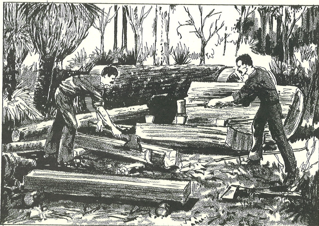
Splitting "billets" from jarrah log and squaring them to make sleepers.
