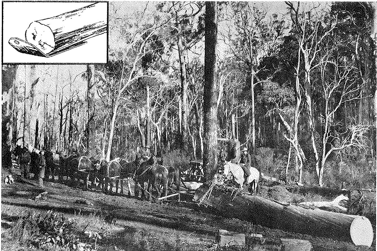
Animal Power: A karri log on two skidders and hauled by bullock team.
