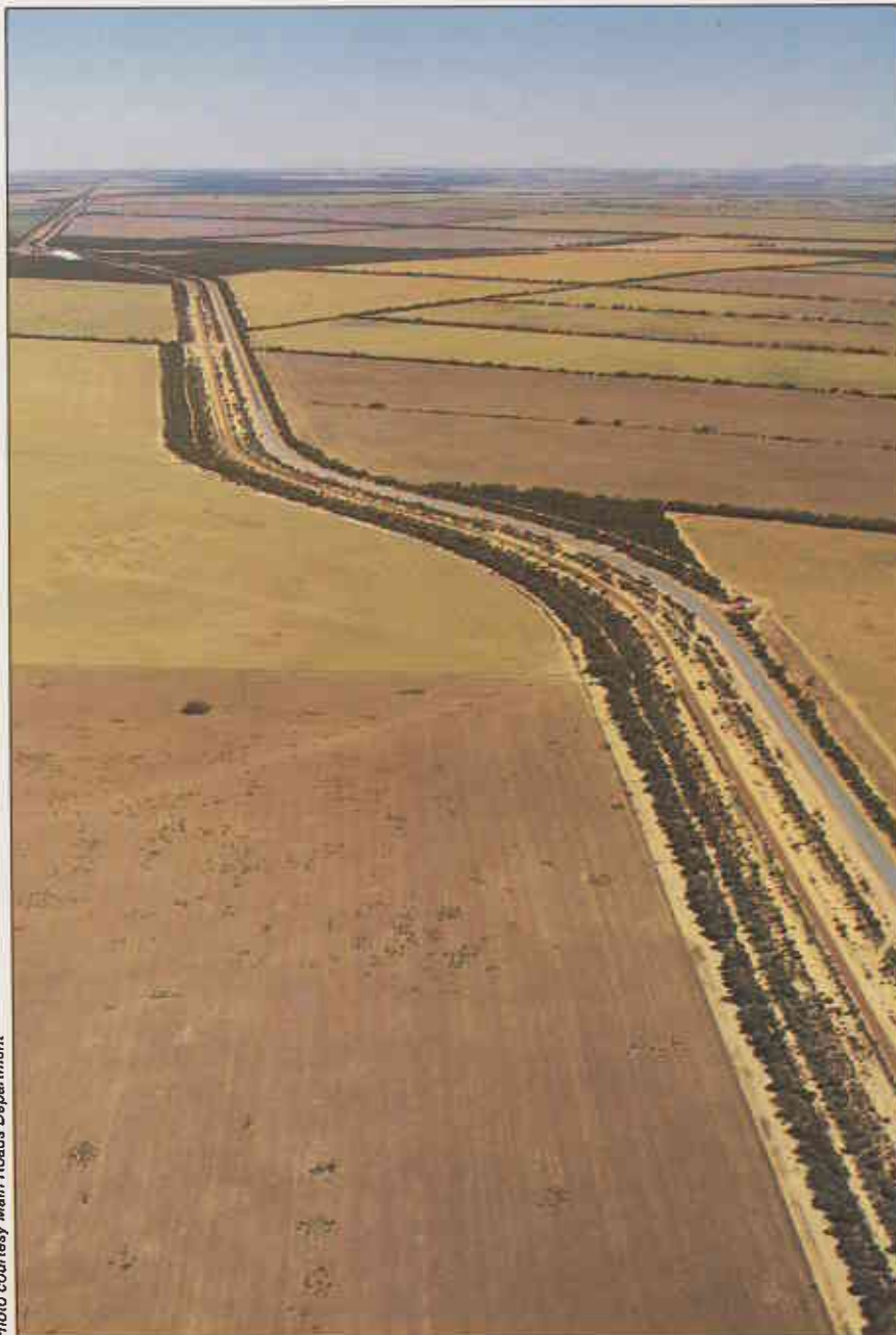
Photo courtesy, Main Roads Department
