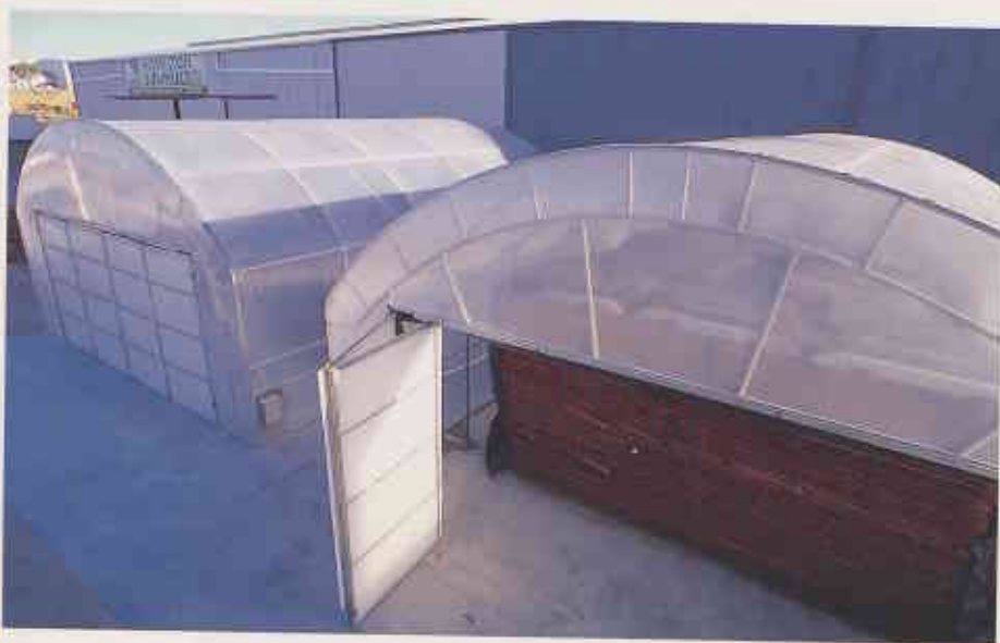
Below: The kiln uses a simple, steel structure, covered with two layers of UV-resistant plastic.
