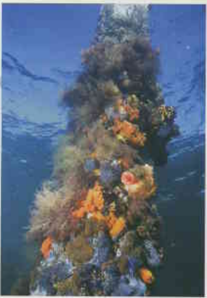
Older piles of the Busselton Jetty are crowded with marine life, but it was not always so. How do marine animals gradually colonise the piles? See page 34.
