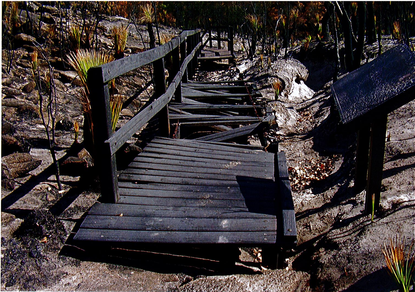
Above Mount Chudalup boardwalk damaged by fire.
