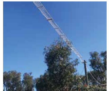
Top left The bridge was constructed at night to minimise disruption to traffic.
