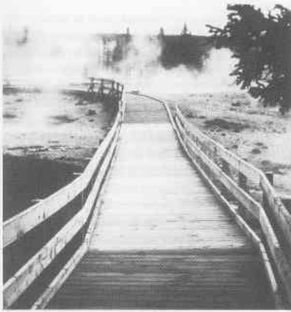
Boardwalks at Yellowstone National Park. Note experimental use of different timber treatments.
