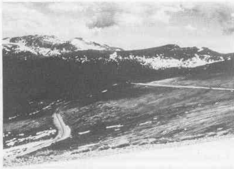
Trail Ridge Road, Rocky Mountain National Park. Note complete lack of guide posts and crash barriers. Only a white line delineates the edge of the road.
