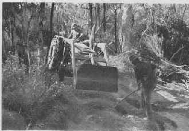
Firebreak construction at Tutanning
