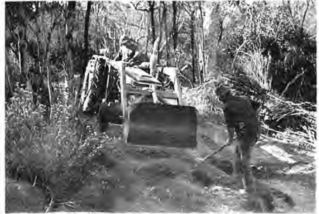
Firebreak construction at Tutanning
