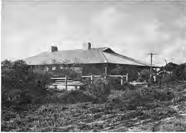
The former Telegraphic Station at Eyre which is now the RAOU Bird Observatory
