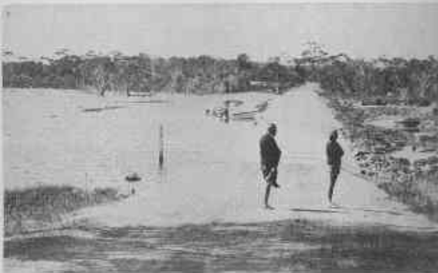
Messrs Aitken and Allen on the weir at Qualandry pool.
