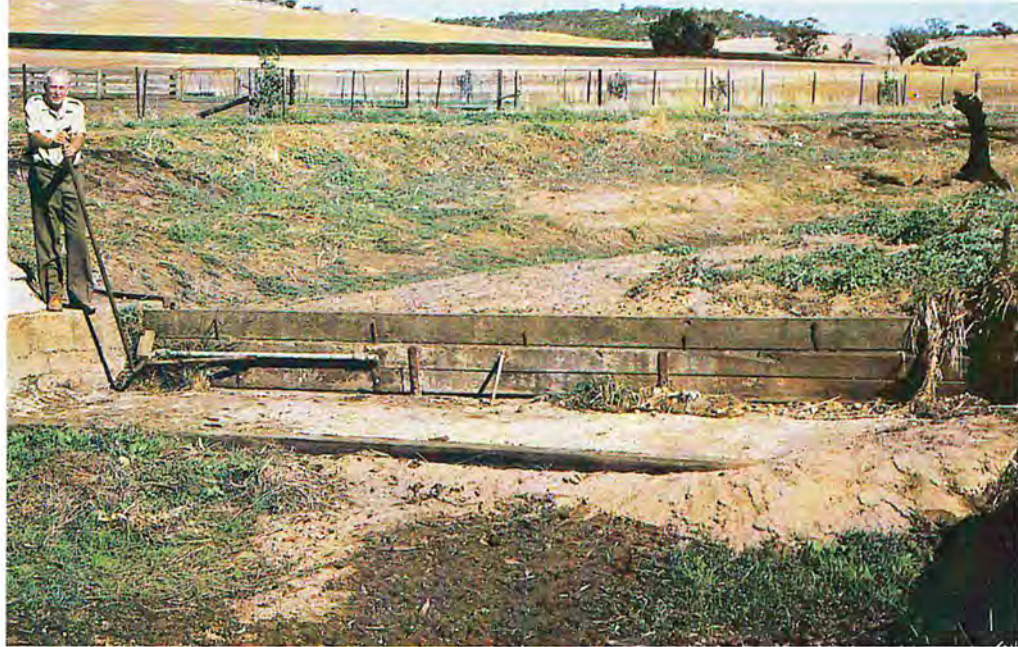
▲ Jim Masters at the controls of one of several simple diversion gates on his property which together control the quantity and quality of water flowing into the farm's dams. This particular gate, when closed, banks up the water level behind it and diverts it into the grill-covered dam inlet (see below). The gate is closed only after any salty surface water has been flushed through.
