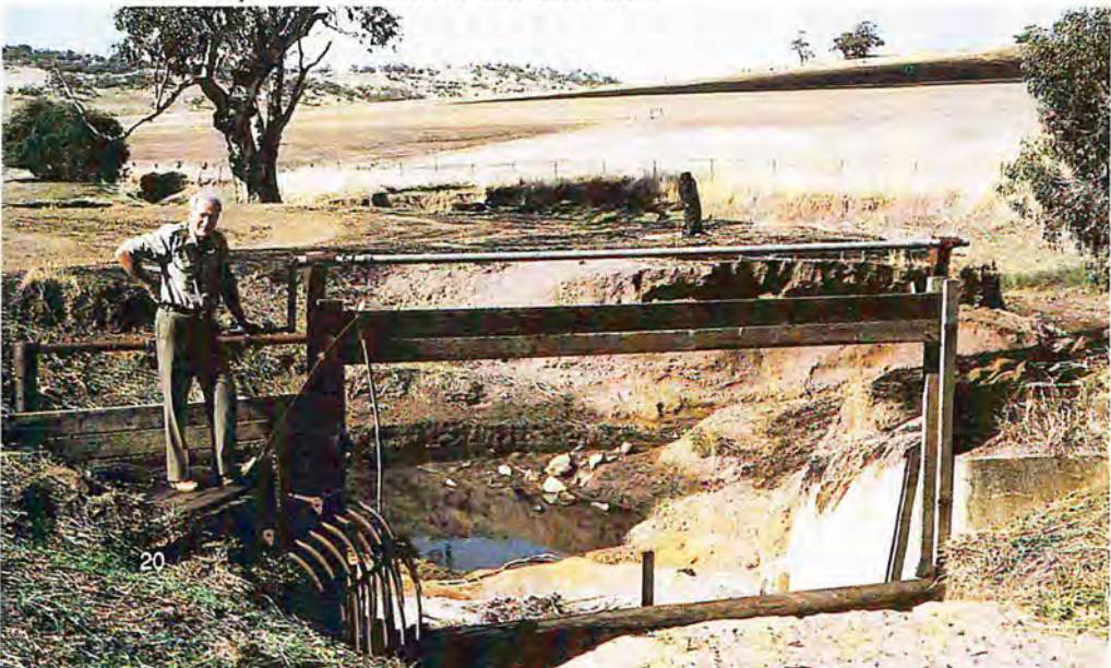
▼ Another diversion gate higher up the watercourse on the same farm as above. Here, the creek is deeper and the water flow faster necessitating different engineering techniques. The planks above the creek are lowered via a crank (left) and the water diverted through the grill on the left to a diversion channel system which takes the water to the dam.
