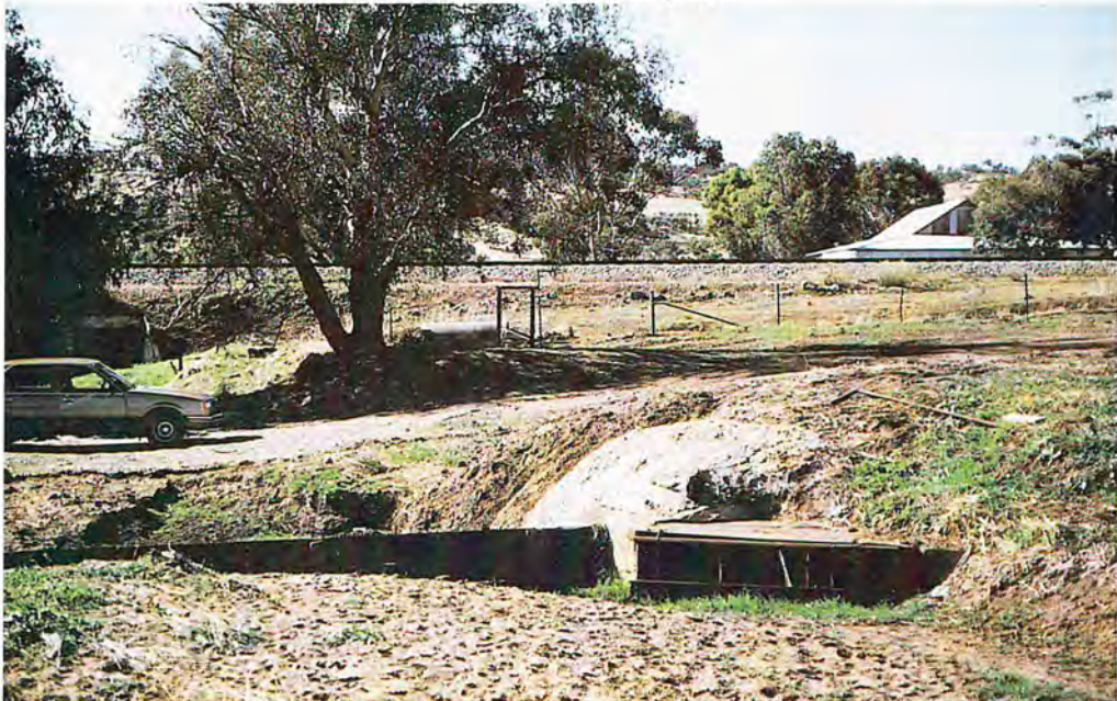
▼ Another diversion gate higher up the watercourse on the same farm as above. Here, the creek is deeper and the water flow faster necessitating different engineering techniques. The planks above the creek are lowered via a crank (left) and the water diverted through the grill on the left to a diversion channel system which takes the water to the dam.
