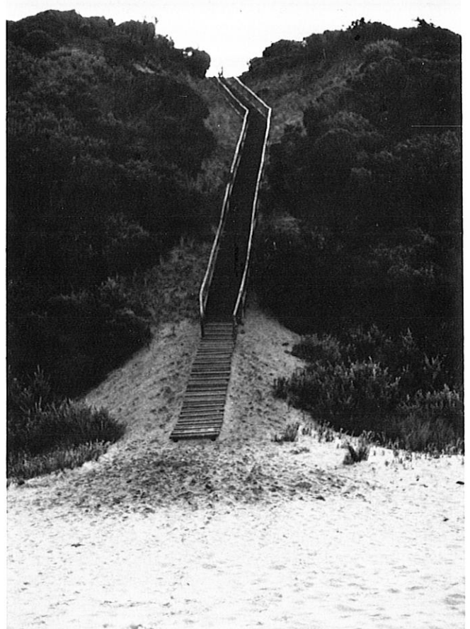
Steps such as these make beach access easier as well as protecting the dune from further erosion. Salmon Holes after new steps project. (Photo: J. Watson)
