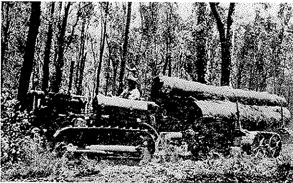
Logging by means of a crawler tractor and Athey Wheel trailer.
