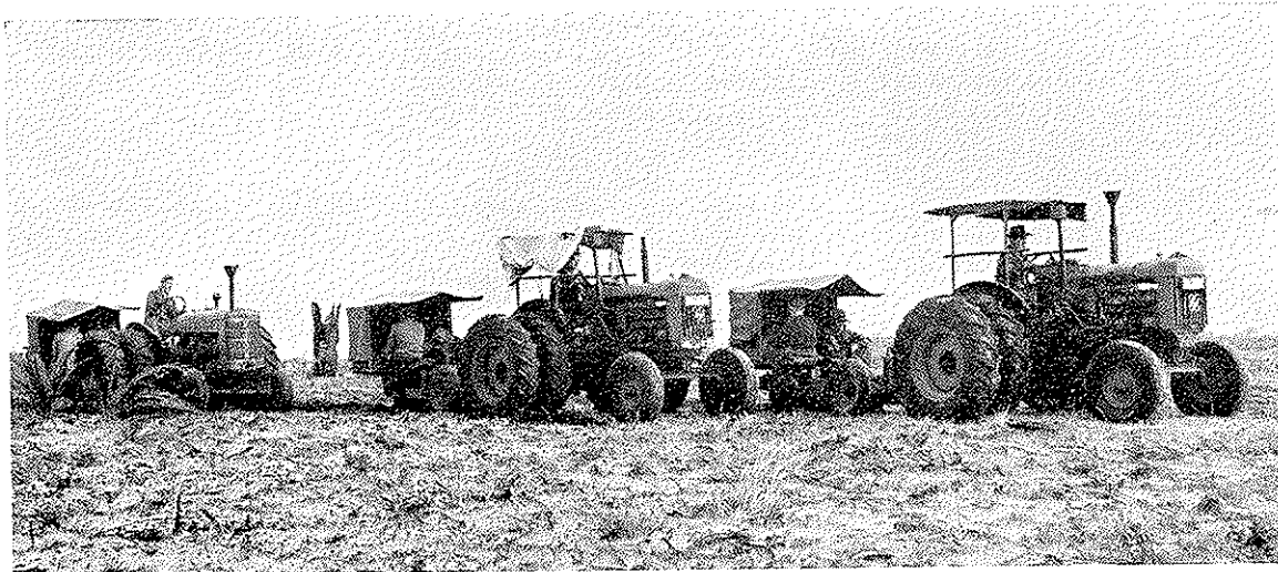
Plate Eleven—Planting Machines in operation on the Coastal area at Gnangara, North of Perth. Machines often work close together in echelon.
