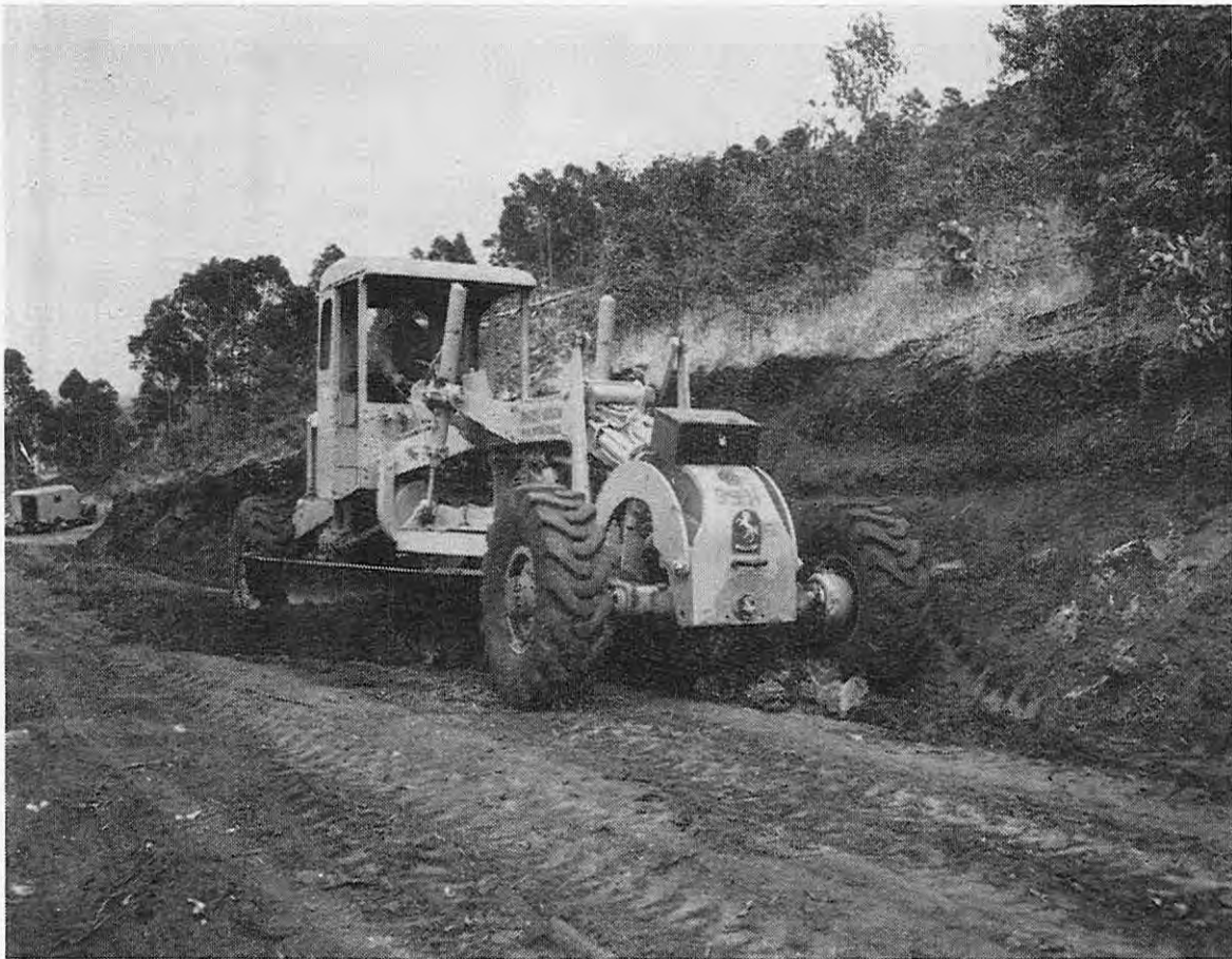
Heavy grader forming road—Blackwood Valley
