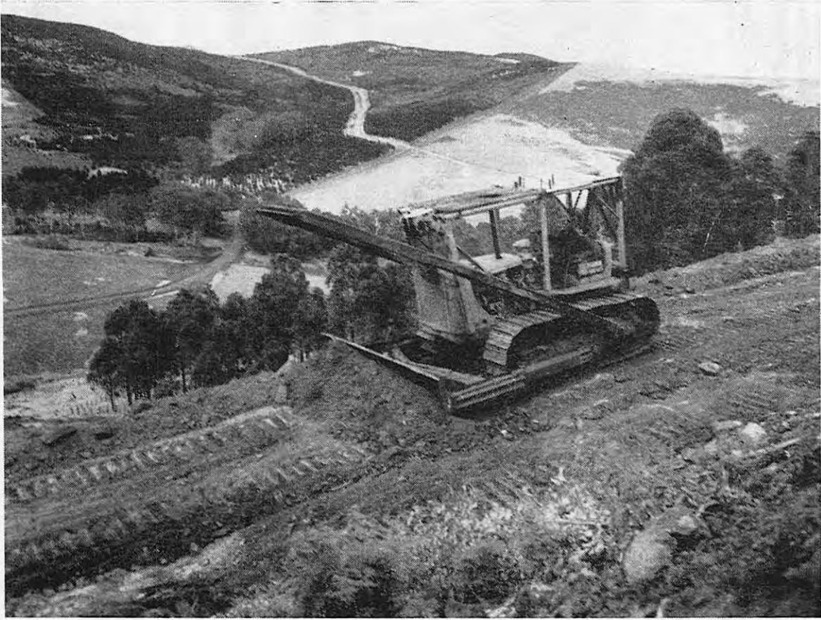
Heavy bulldozer constructing road—Blackwood Valley
