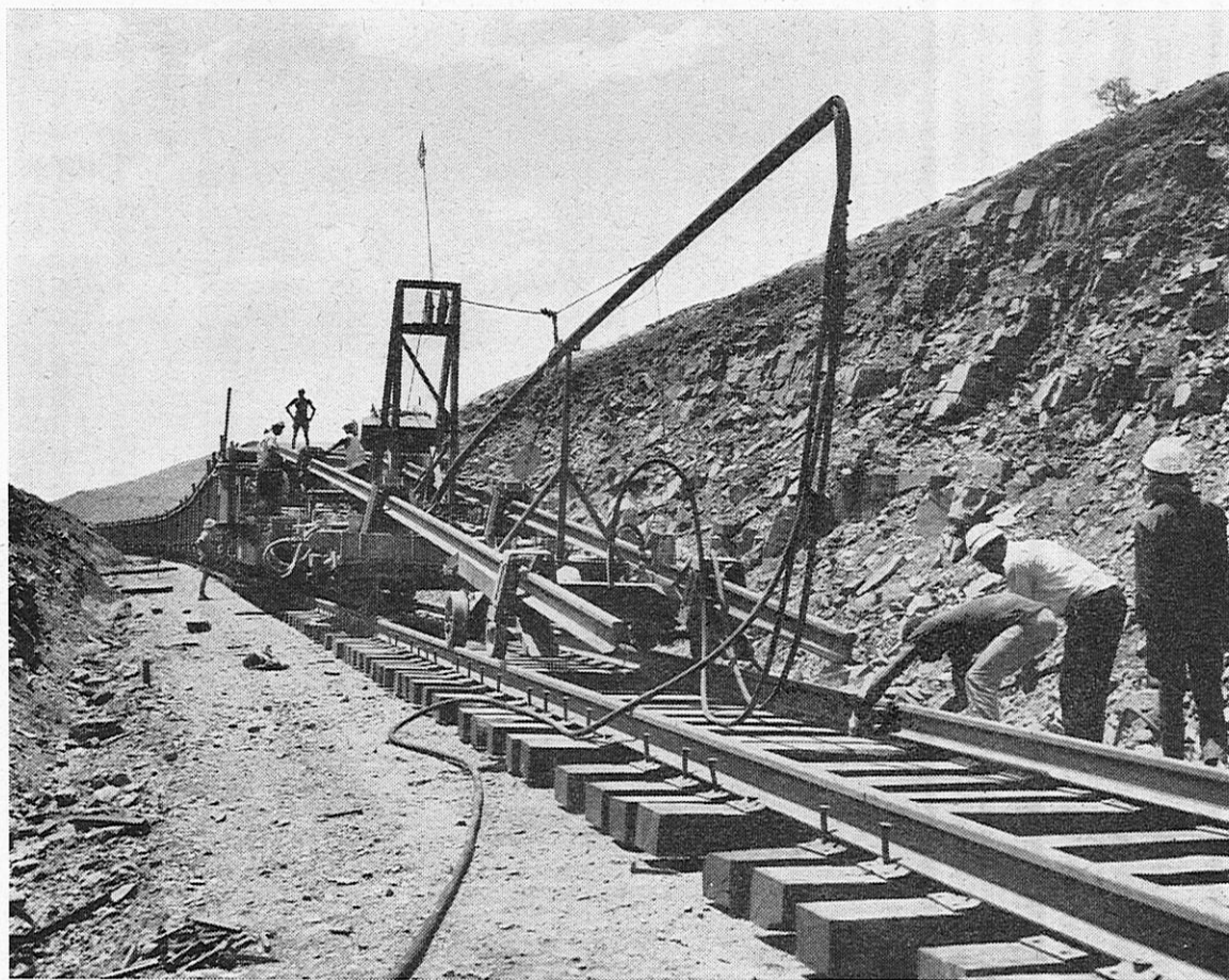
Track-laying for the Hamersley Iron railway line.
