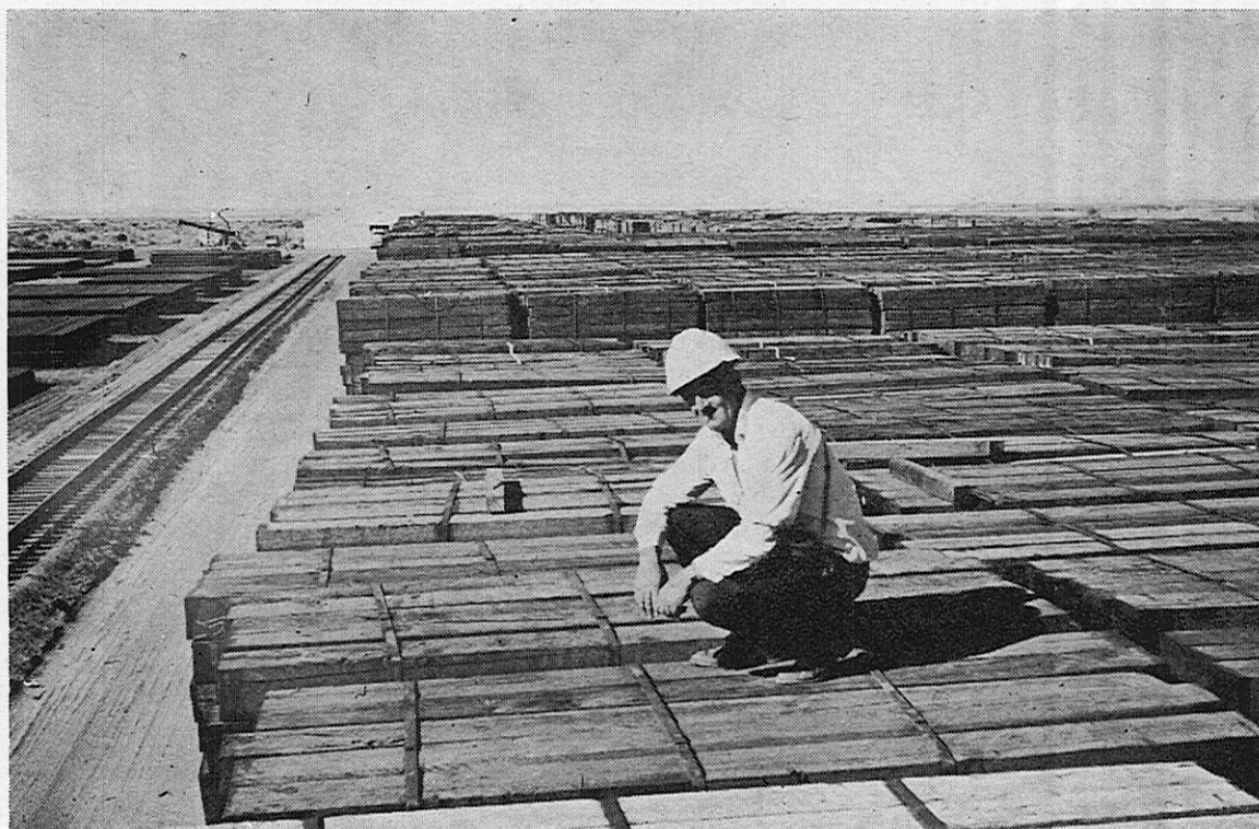
Some 290,000 railway sleepers, 8ft. 6 in. long x 9 in. x 6 in., mostly jarrah with some wandoo and yarri, stockpiled at the Port Hedland depot of Mt. Newman Co. Nearly three times this number will be needed to complete the 280 miles of railway line between the iron-ore deposits of Mt. Newman and Port Hedland.
