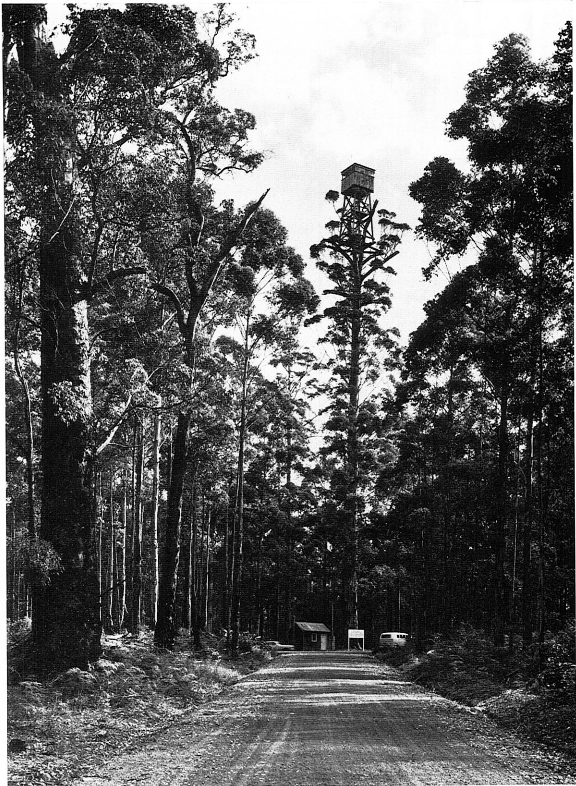
The famous Diamond Tree fire lookout. To obtain a clear view over the surrounding forest, a 20 feet wooden tower was built 160 feet above ground level in the branches of a karri tree—note the karri regrowth nearby. First manned in 1942 the lookout is situated only a few chains off the South-West Highway about six miles south of Manjimup.
