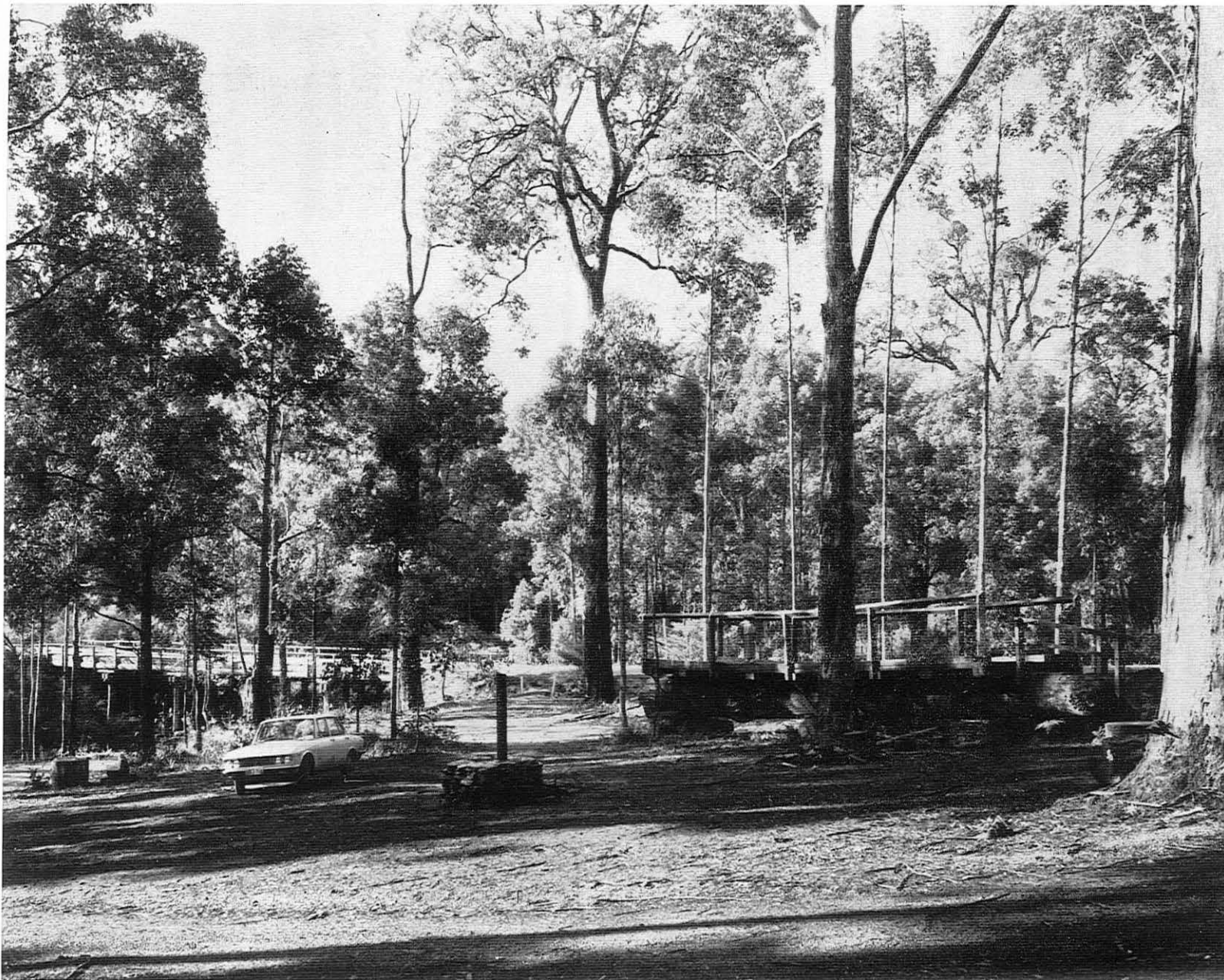
Above—One Tree Bridge picnic spot on the Donnelly River west of Manjimup (1972). In 1904 a karri tree was felled across the stream to provide the basis for a bridge serving the nearby graphite mine. The bridge remained in service until 1943.
