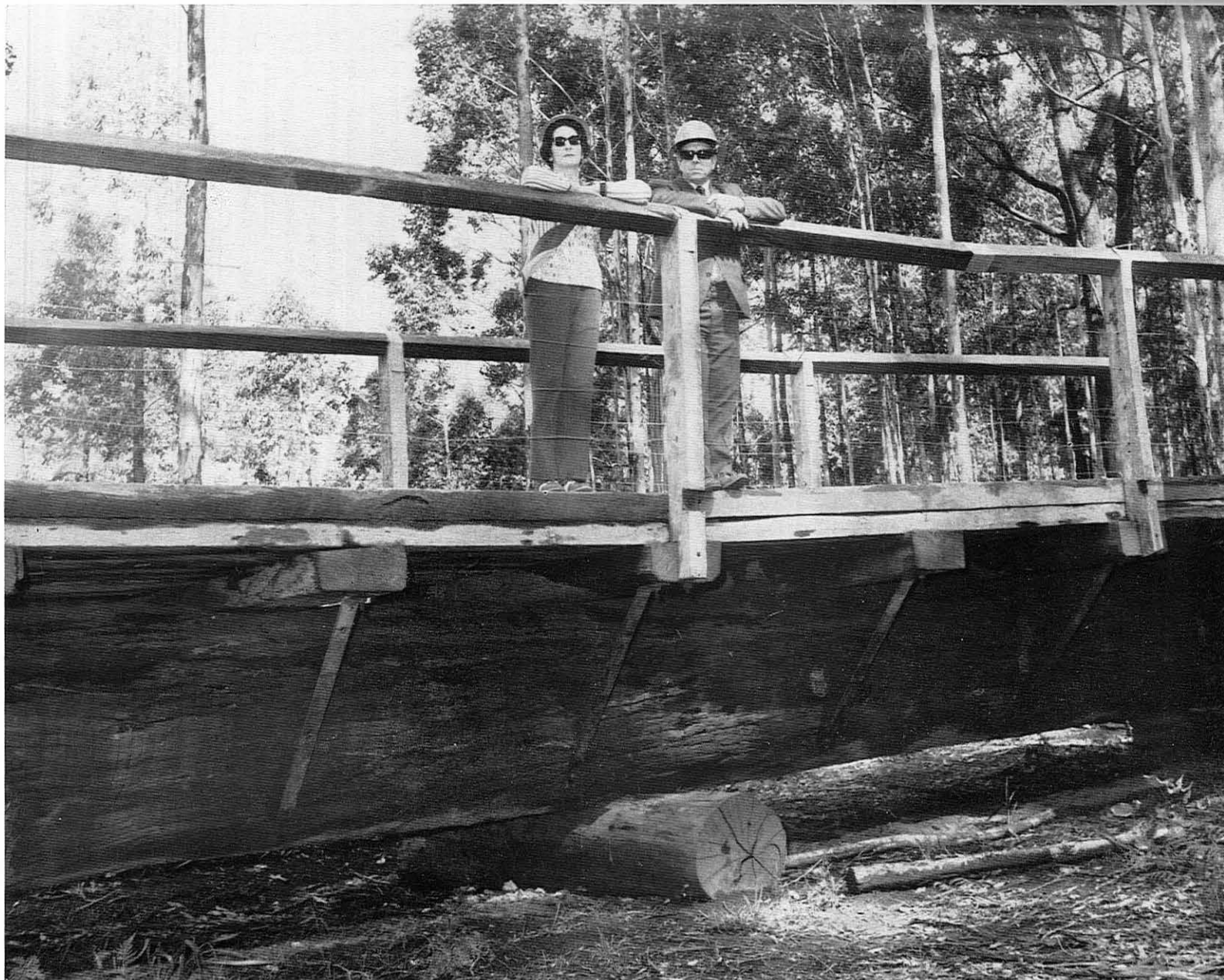
Above—In 1971 a section of the old bridge was recovered from the river and reconstructed on the bank nearby (photograph—1972).
