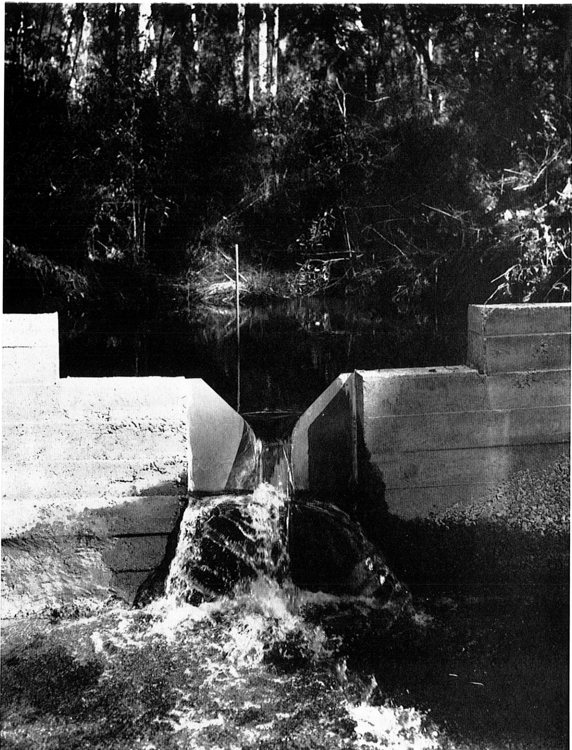
Notch-weir stream gauge south-east of Manjimup.
