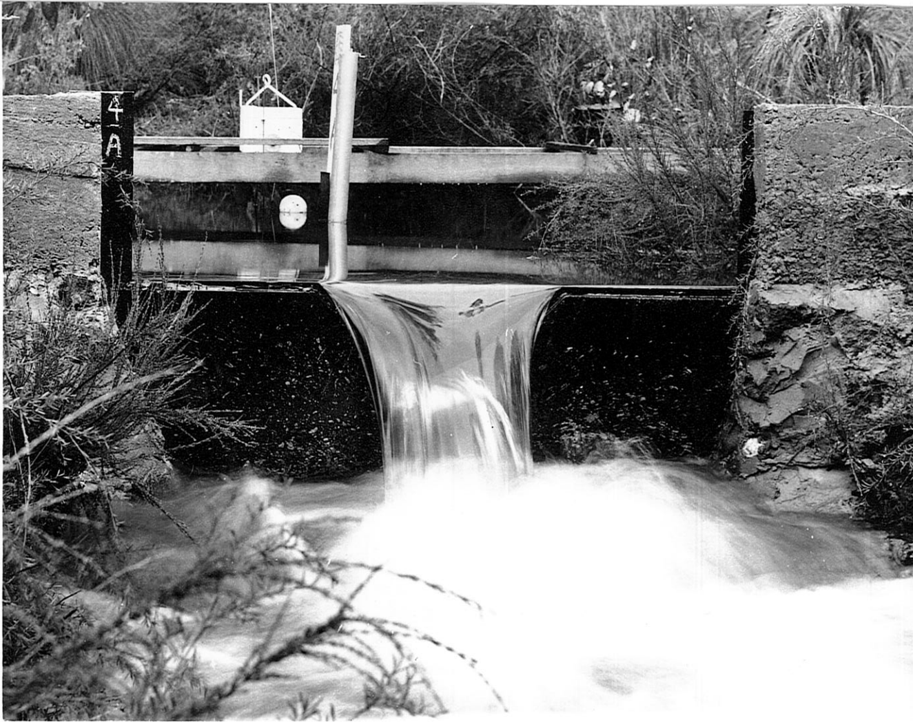
Fig. 3 Combination "V" notch weir constructed by Dwellingup gang.
