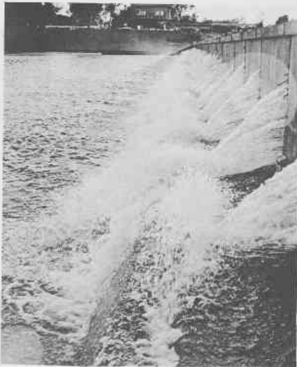
Photo 5. Fitzroy Barrage - Far-side (R.H.S.) Showing Apron
