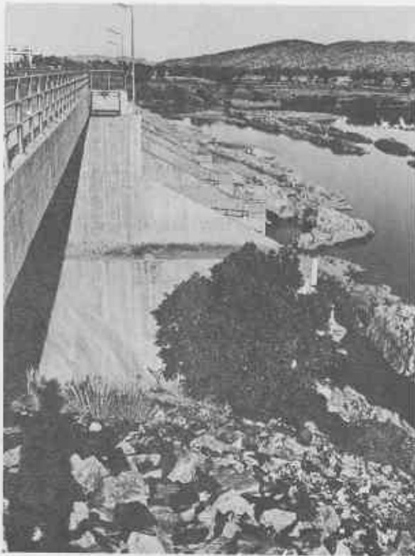
Photo. 12. Ord River Diversion Dam. Kununurra or Left-hand Side Site for Fishway
