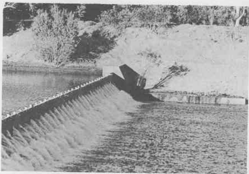
Photo. 7. Fitzroy Barrage - Far or Right-hand Side Site for Fishway
