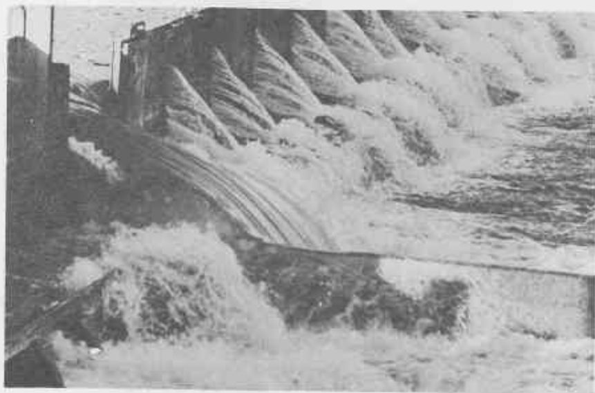
Photo. 4. Fitzroy Barrage - Spill of Water over a Collapsed Automatic Gate
