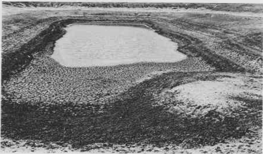
Leeman's Dam Near Westonia.
