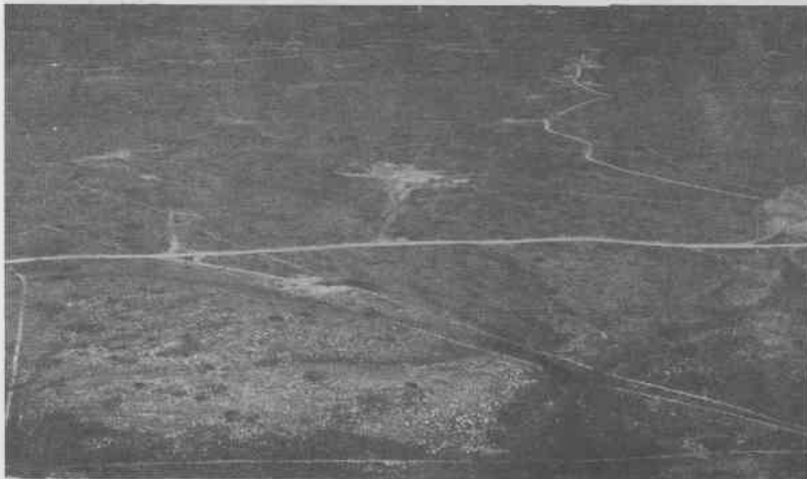
Plate 4. General view of oilfield.
