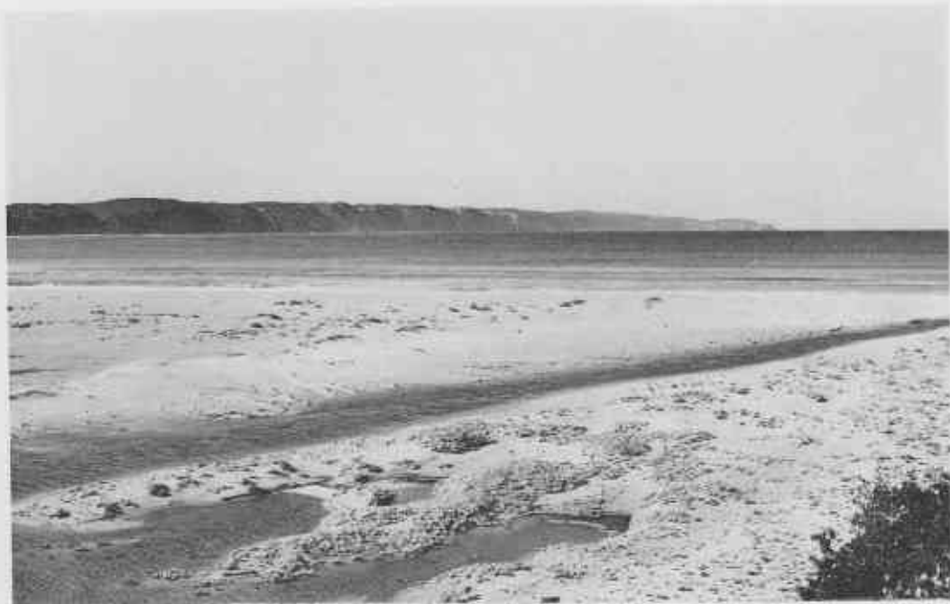
Plate 1—The first step in the opening of the estuary. A channel has been bulldozed from the estuary to the centre of the sand bar, a week or so prior to the opening date.
