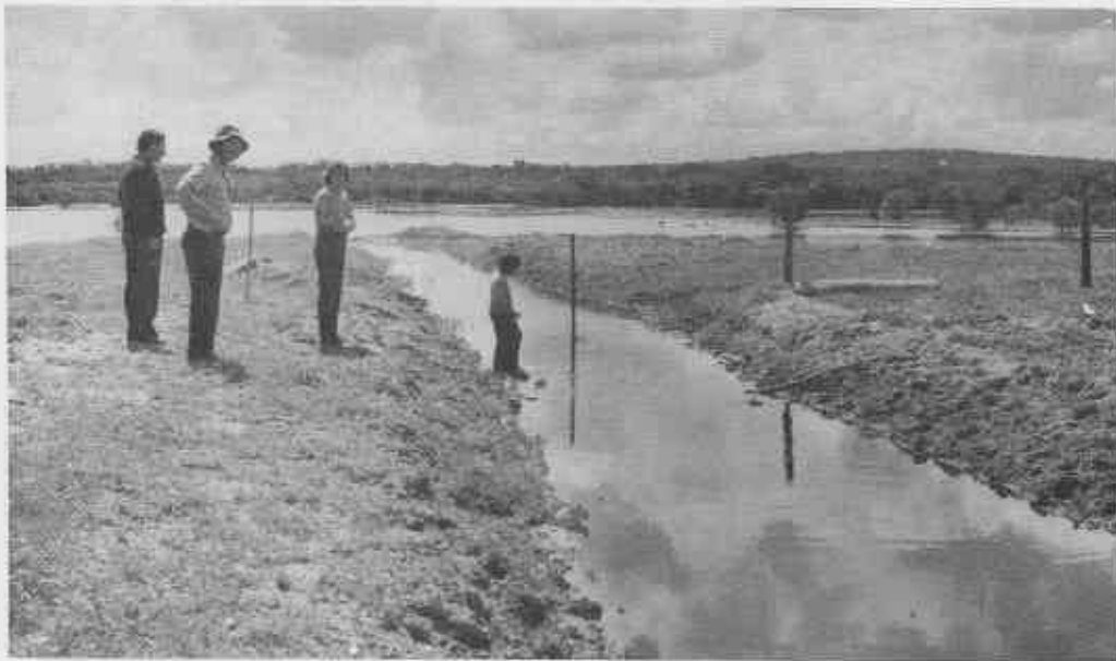
10. Southern drain dug in the early 1970's. (Photo: A. Fewster)
