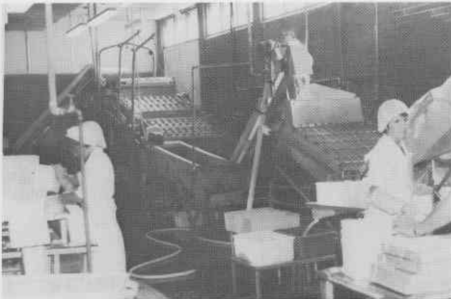
PLATE 16: THE AUTOMATIC PRAWN PEELING MACHINE.
