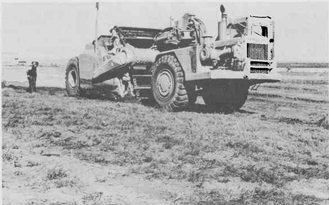
PLATE 2. Subsequent removal of topsoil to an average depth of 15 cm by an elevating scraper prior to mining. Topsoil so collected is either stockpiled for later use or used immediately for rehabilitation.
